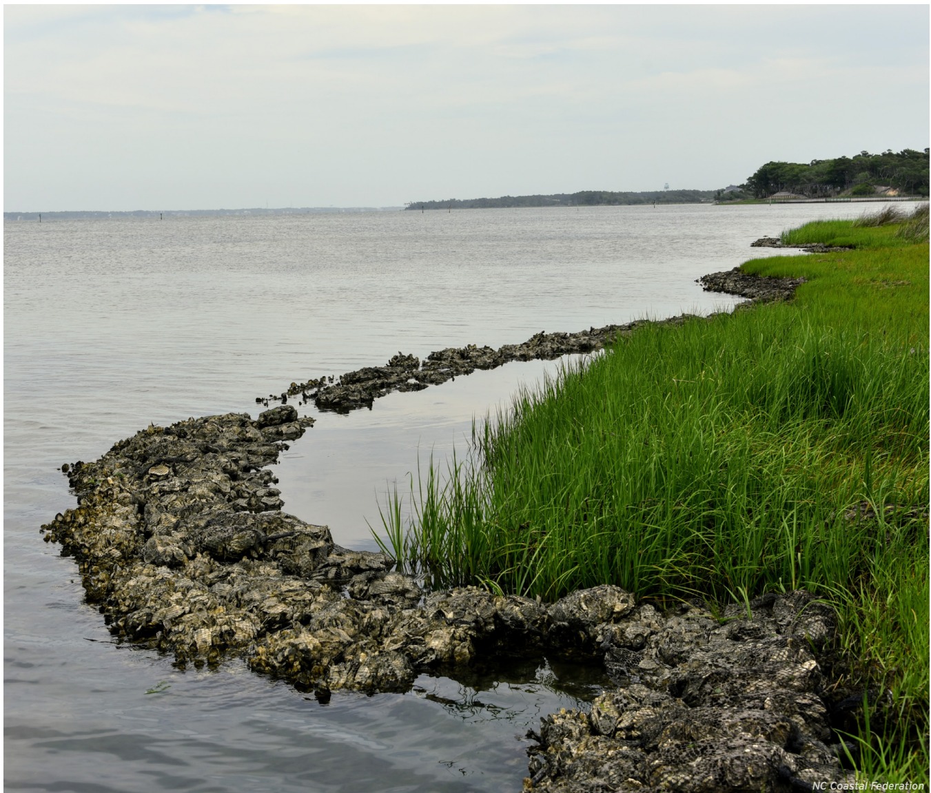
Shoreline Restoration Project with Salt Marsh Plugs and Oyster Shell in Bogue Sound
